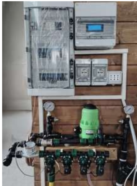
Fig. 3. Front view of the central unit in standalone configuration with integrated pump. Top: logic panel with microcontroller, power supply, and relay system. Bottom: hydraulic manifold with zone solenoid valves, pressure gauges, and impulse water meter.
