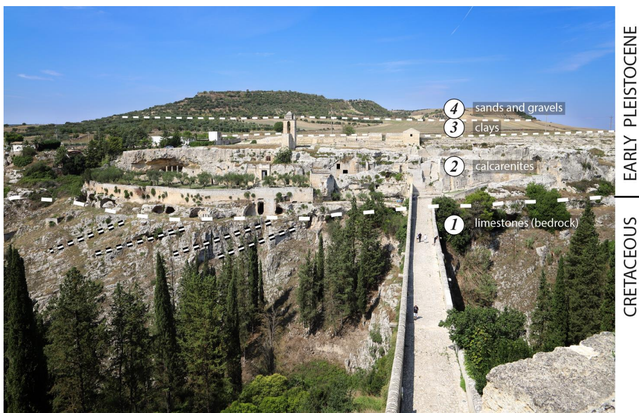
Figure 8. The thin Bradanic Trough (foredeep) succession along the Gravina (canyon) of Gravina in Puglia town, at the toe of Murge. After having eroded the Quaternary foredeep succession, the stream cut the bedrock, made up of Cretaceous limestones. Note the angular unconformity between tilted Cretaceous strata and the overlying sub-horizontal younger sedimentary units. Photo by D. Belfiore [77].
