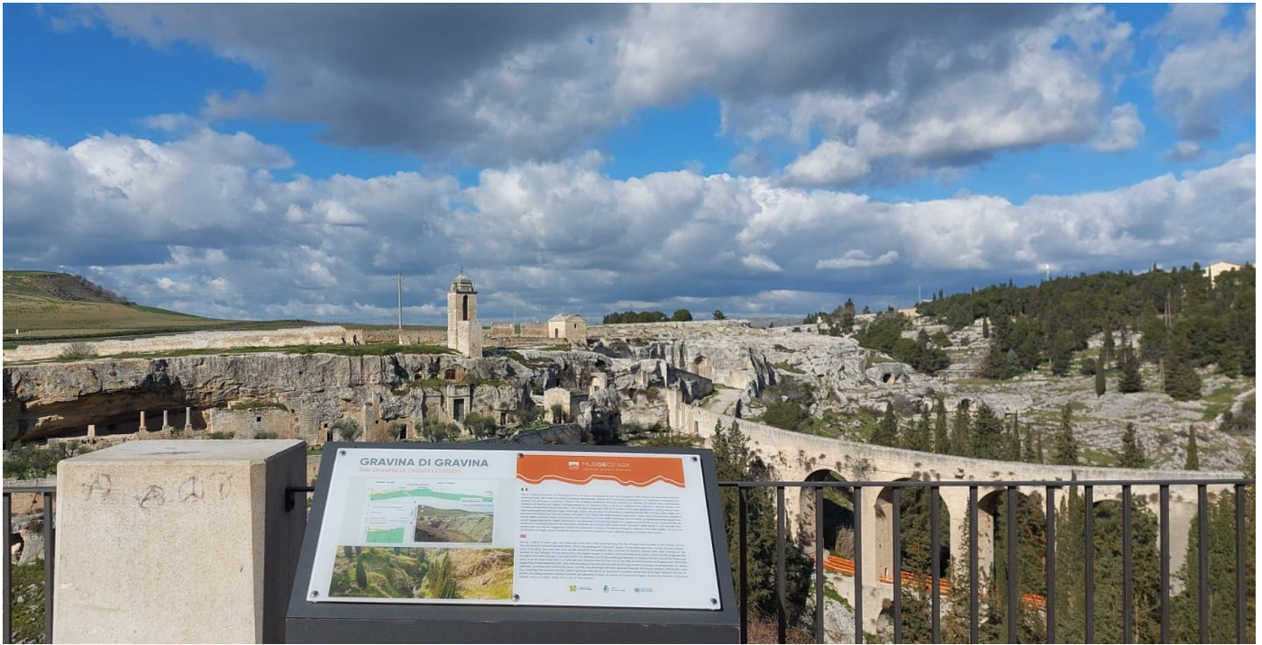
Figure 12. The Aqueduct Sant’Angelo—Fontana della Stella (corresponding to the bridge at Gravina in Puglia town). Note the explanatory panel in front of the panoramic point. Photo courtesy of Giusy Schiuma.
