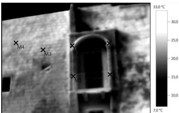
Fig. 6 Thermographic relief of a section of church wall S
