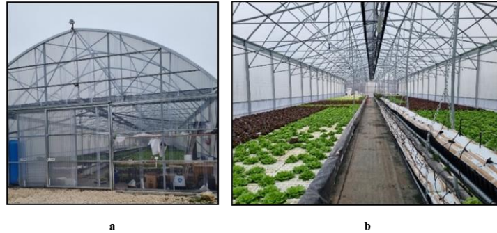
Fig. 1. Hydroponic greenhouse structure pictures; a. external environment; b. indoor cultivation environment.
