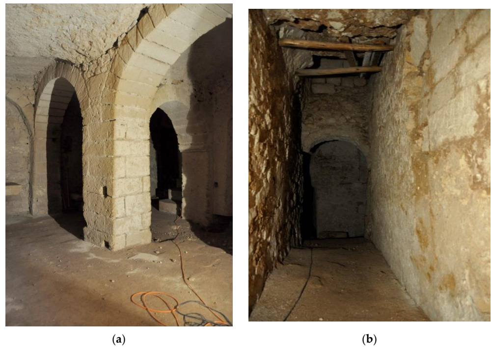
Figure 7. (a) View of the aisles; (b) View of the corridor.
