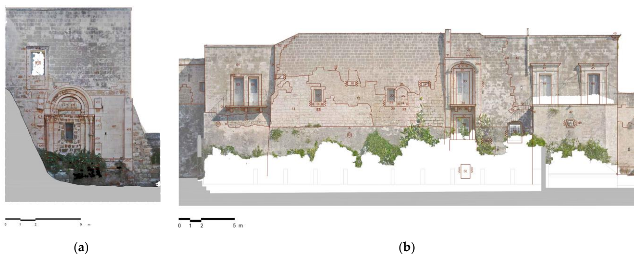
Figure 19. Stratigraphic analysis of the façade: (a) Western façade; (b) Southern façade.
